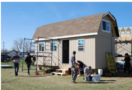
Tiny home project in progress at Kainai High School
